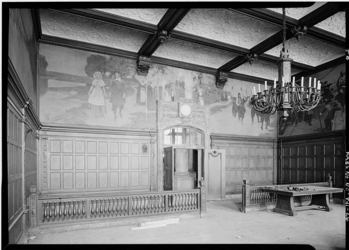
Archival photograph (overall) of water damage
